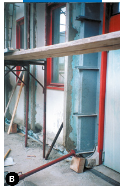
Repair of damaged precast panel "ribs" with concrete manufactured with Stabilcem SCC. A - Before repair. B - After repair.
