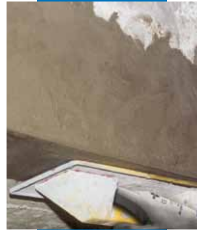
Patch-work of a concrete beam
