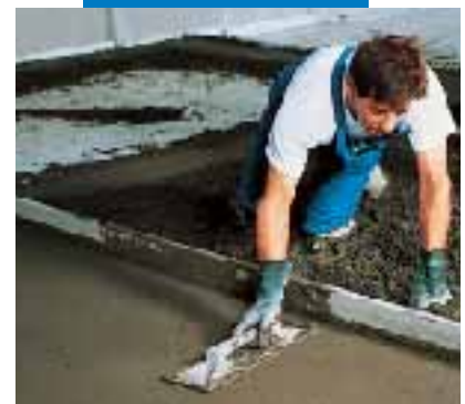
Tamping the Mapecem screed
