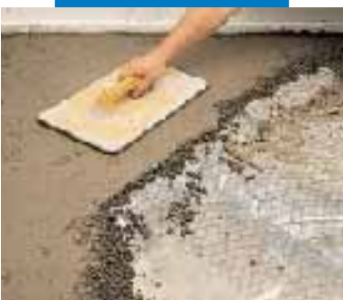
Covering pipes with Mapecem and reinforcement netting
