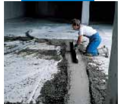
Preparing a levelling strip
