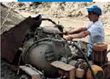
Mixing Mapecem with an automatic pumping unit
