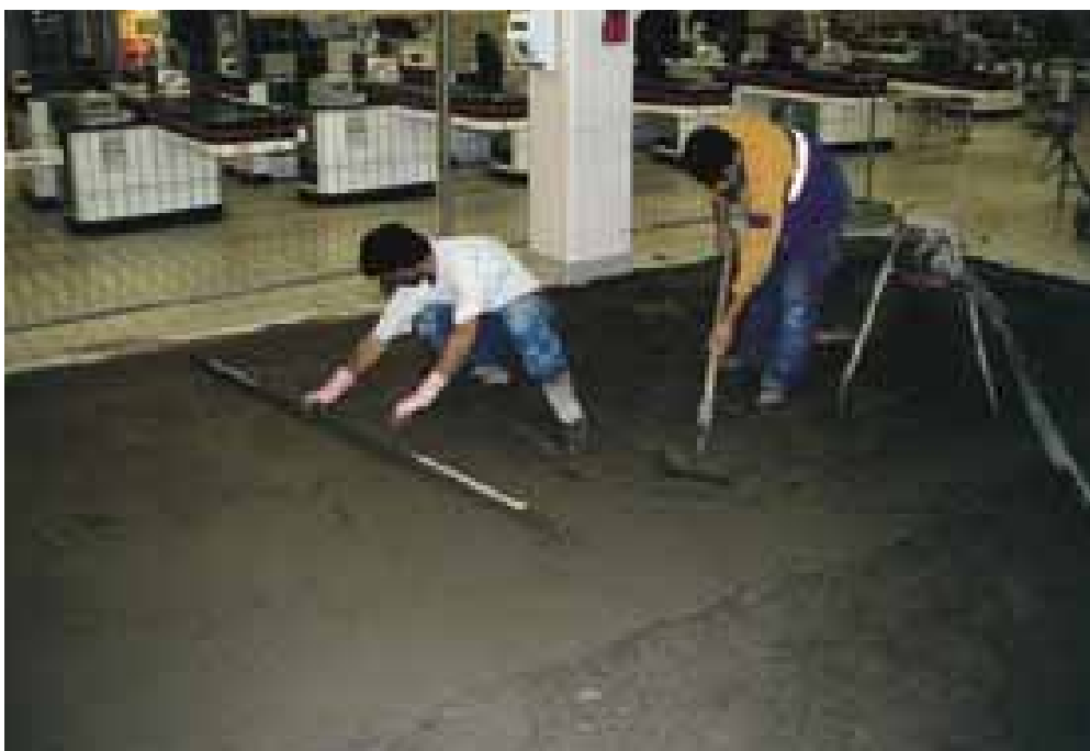
Fast repair of a screed in a supermarket
