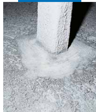
Column waterproofed with Idrosilex
