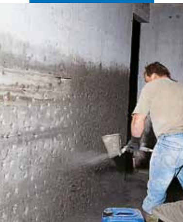
Spraying on the first coat of mortar admixed with Idrosilex Liquid
